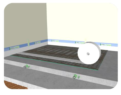
Laythe anti-pitting coat on the surface of the lightened screed, once cleaned from various debris from previous work. The cover should be laid with edges well placed and cut as close as possible to the outer edge, so as to avoid dangerous acoustic bridges. Once the acoustic coating is installed on the entire surface to be treated, all joints must be uniformly sealed with **ROTOCELL AD** adhesive strip.
