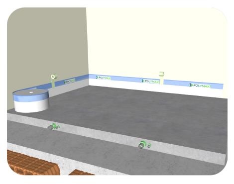
Apply the adhesive part of the **POLYBAND AD** desolarizing tape, removing the protective foil, at the base of the wall and support with some pieces of tape the protective nylon that must be laid on top of the radiant panel. The strip is laid with the shorter side of the nylon-strip fastening towards the lightened screed. This application must be carried out continuously on the entire perimeter of the rooms to be treated.
